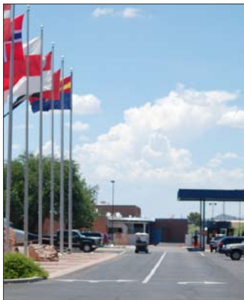
During construction, traffic to the east side of the base will enter through the Main Gate and this one-way street will temporarily service two-way traffic.
