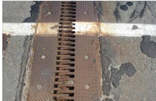
Non-Bicycle Compatible Bridge Expansion Joint
