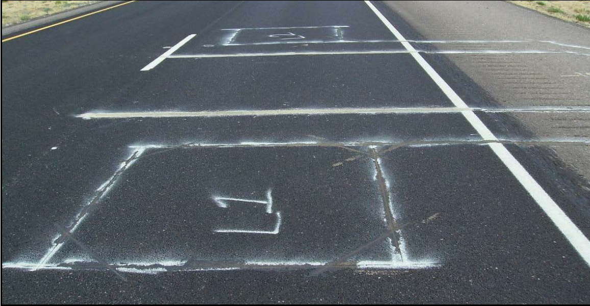
Figure 4. Photo. In-line weigh sensors (quartz piezos) and detection loops (double threshold system).
