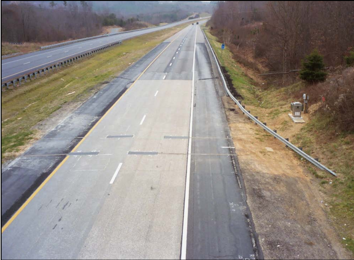
Figure 7. Photo. Two-lane WIM site, with Portland cement concrete (PCC) pavement installed for approach and departure.
