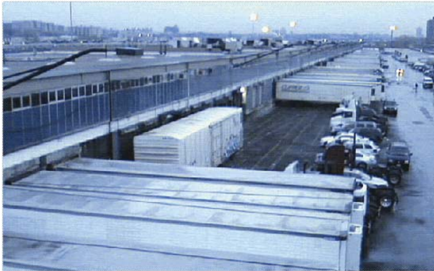
Figure 4.3 When Truck and Rail Access Are Not Separated, Inefficiencies (Such as the Orphaned Railcar Shown, Center) Can Impact Operations
