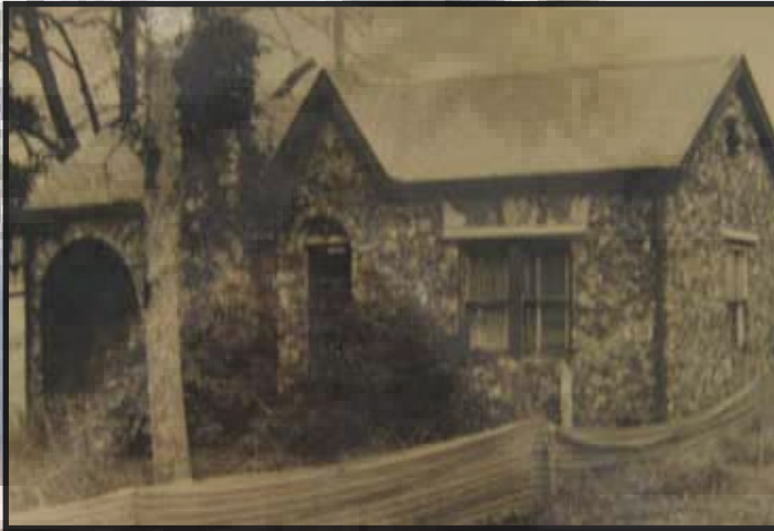
Pictured is the Bankston House in 1993, before rehabilitation. Renovation took place in 2000 and restored interior and exterior architectural features including the exterior stonework, doors, windows, fireplace, floors and ceilings. In addition to modernizing existing office space, the side and back porches were enclosed to create more usable space. Mission-style furniture purchased through the General Services Agency (GSA) creates a 1930s-style décor. The Environmental Flight now uses the house as administrative office space to manage the Dobbins ARB environmental protection, pollution prevention and natural/cultural resources programs. (U.S. Air Force courtesy photo)
