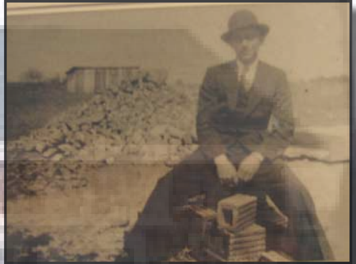
J.C. Bankston Jr. sits atop the hollow-core tile blocks used for the interior and exterior walls of the house. The structure in the background is the outhouse that served the residence already on the property purchased by J.C. Bankston Sr. (U.S. Air Force courtesy photo)
