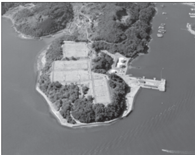
An aerial view of Defense Fuel Support Point Iorizaki, Japan. (Courtesy photo)
