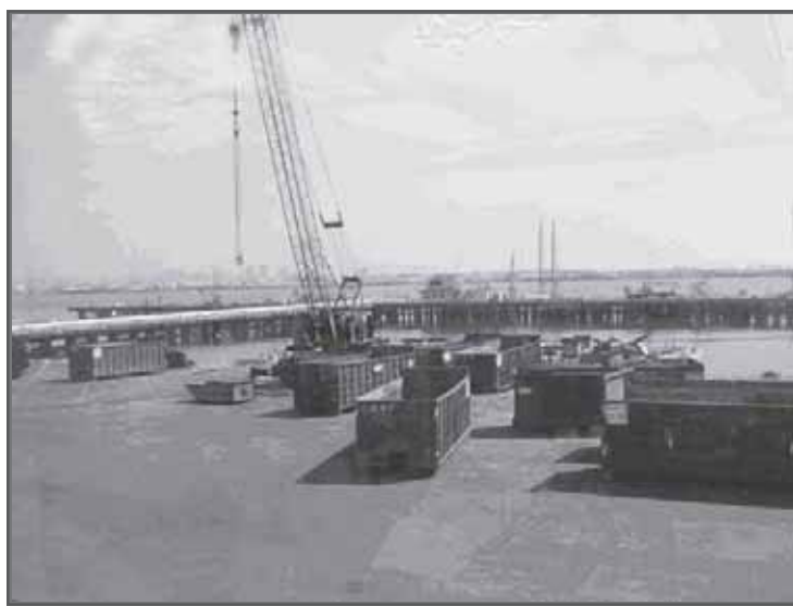
Repairs to the pier are underway. (Photo by Steve Frey)
