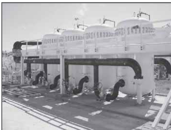
DESC clay filtration vessels at the Las Vegas terminal Kinder Morgan facility outside of Nellis Air Force Base, Nev. (All facility photos by Lt. Col. Jon Ramer)
