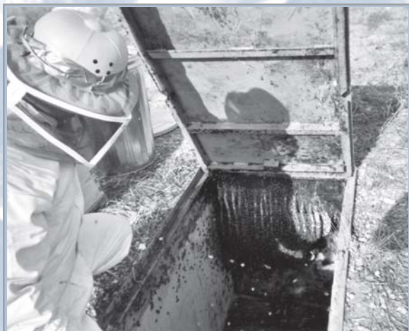
John Rifalato, DFSP superintendent, peers into a conduit box in which wild bees have built a hive. Rifalato and his team were transferring the bees to wooden hives for domestication.
