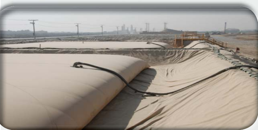
Fuel bladder used in the Middle East. Photo by DLA Energy Middle East.
