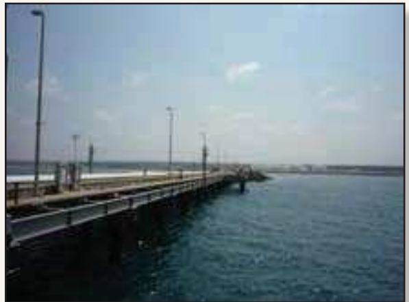
Pierside fuel facilities at the Horizon Terminal contractor-owned-and-operated Defense Fuel Support Point Djibouti, which provides fuel to U.S. Naval vessels transiting the Suez Canal.
