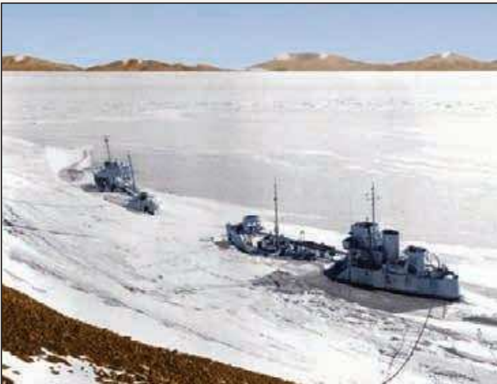
Two U.S. Navy Yard Oiler Ships lie frozen into the annual sea-ice at the McMurdo Station construction site in 1956. These were used as fuel storage facilities while the base was being built. National Science Foundation photo by Navy Cmdr. Jim Waldron.
