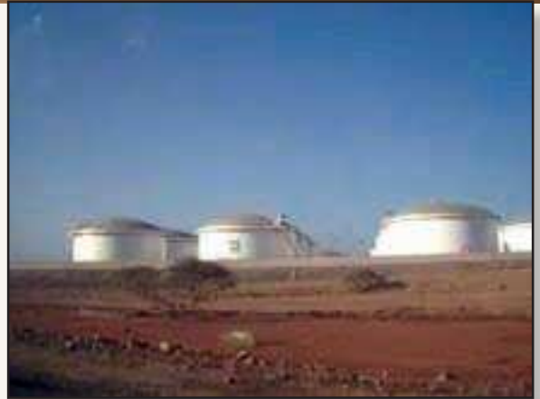
Fuel storage tanks at the Horizon Terminal contractor-owned-and-operated Defense Fuel Support Point Djibouti. The Defense Logistics Agency-fueled DFSP provides fuel to U.S. Naval vessels transiting the Suez Canal.
