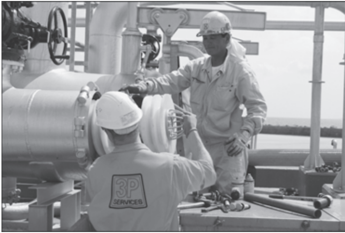
A scrubber pig launched by contractors Weston Solutions and 3P starts the 505th Quartermaster Battalion's pigging operations on Okinawa in August.
