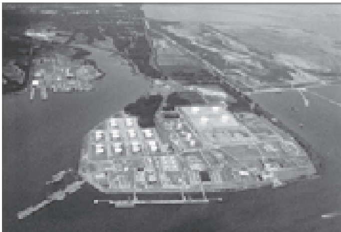
Defense Fuel Support Point Craney Island, Va., is one of 627 the Defense Energy Support Center's DFSP Management directorate oversees.
