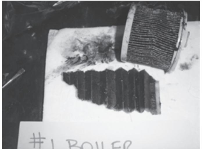
Below: This photo is of the ship-service boiler filter. The small gel-like globules are clearly present, said Coast Guard Lt. Miles Randall.
