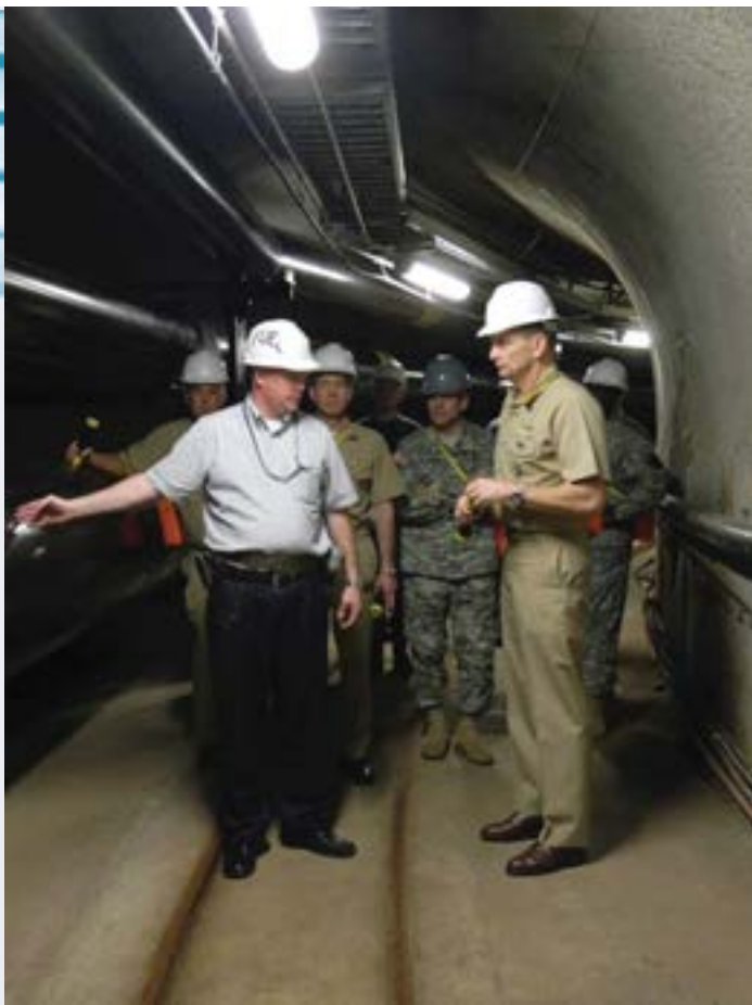
Navy Vice Adm. Mark Harnitchek was briefed on and had a tour of the Red Hill underground fuel storage facility. The facility consists of 20 fuel tanks located hundreds of feet below ground and was constructed between 1940 and 1943 to replace vulnerable above-ground fuel storage tanks that were located around Pearl Harbor. Photo by Monique Randolph.
