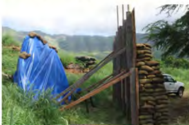
Petroglyphs protected with barrier during detonation of unexploded ordnance
