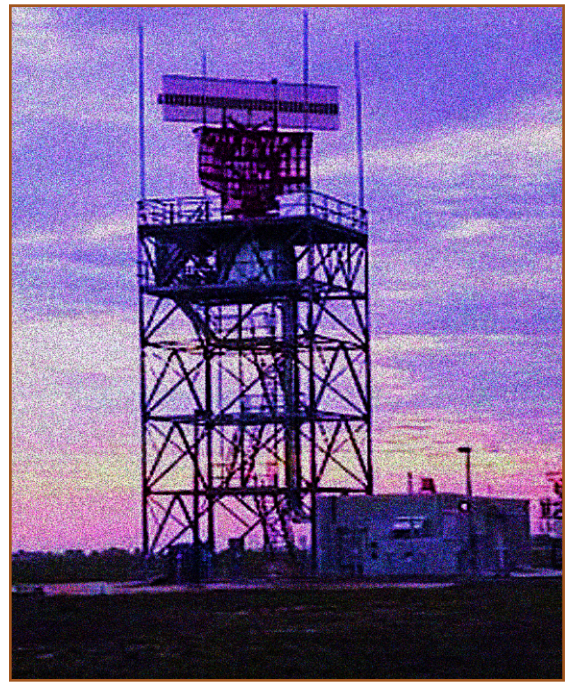
A Digital Airport Surveillance Radar (DASR) antenna.
