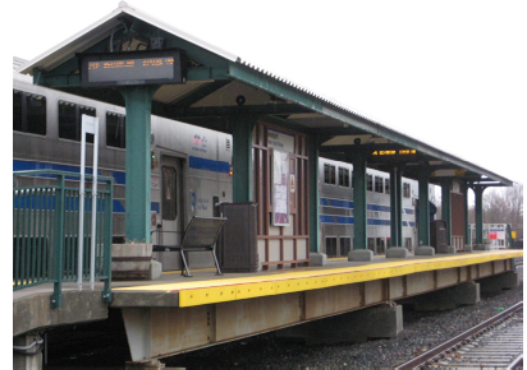
A typical Long Island Rail Road commuter rail platform, Southold Station. (Volpe Center Image)
