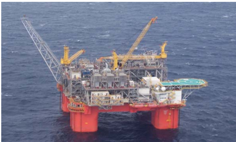
Atlantis, is a floating oil and gas production facility operated by British Petroleum in the Gulf of Mexico and the site of an ADS-B VHF Communication Radio Transceiver as well as an Automated Weather Observation System Station. (Volpe Center photo)
