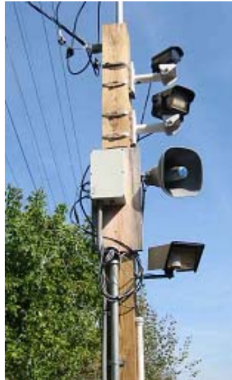
A trespass detection and deterrent system installed on a railroad bridge in Pittsford, New York. This equipment allows railroad security to remotely monitor ROW and respond to incidents effectively. (Volpe Center photos)
