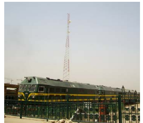
Baghdad Central Station with microwave tower in background. The COI is helping rebuild Iraqi infrastructure in support of DoD and DOS. (Photo courtesy of Mafeks International, LLC)
