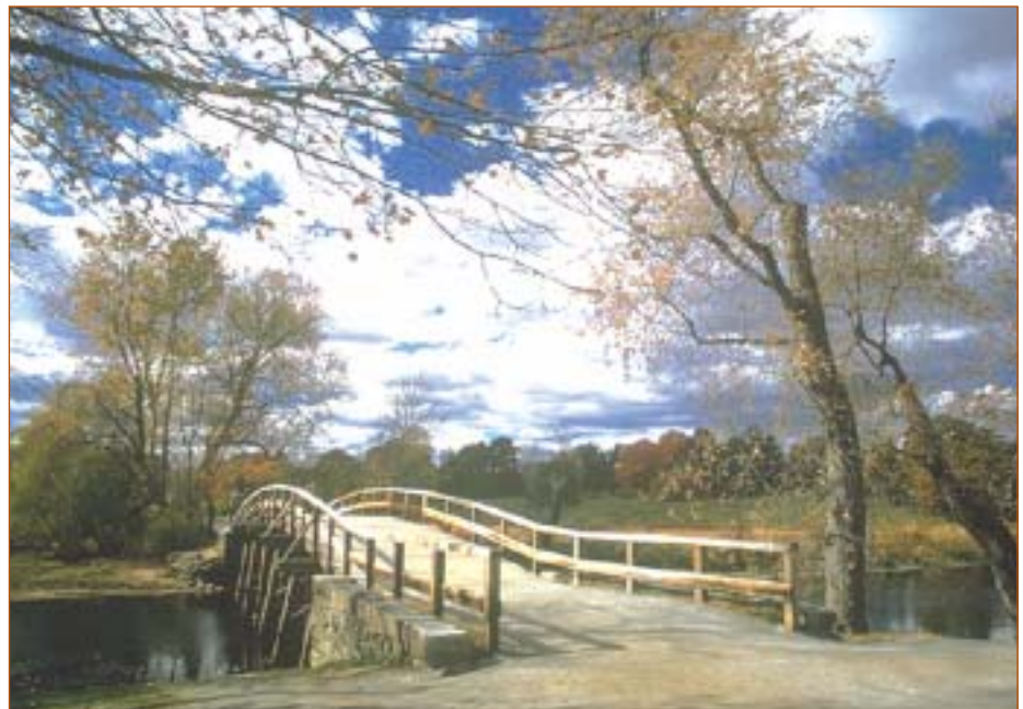
North Bridge in Minute Man National Historical Park in Concord, Mass., is the site of the "shot heard 'round the world" and the opening battle of the American Revolution. Important historic sites such as this can be jeopardized by the effects of increased vehicle traffic in and around national parks. The Volpe Center is actively engaged in NPS efforts to provide efficient park access while preserving natural and cultural resources for future generations. Projects range from individual park traffic studies to a system-wide transportation plan. (NPS photo)
