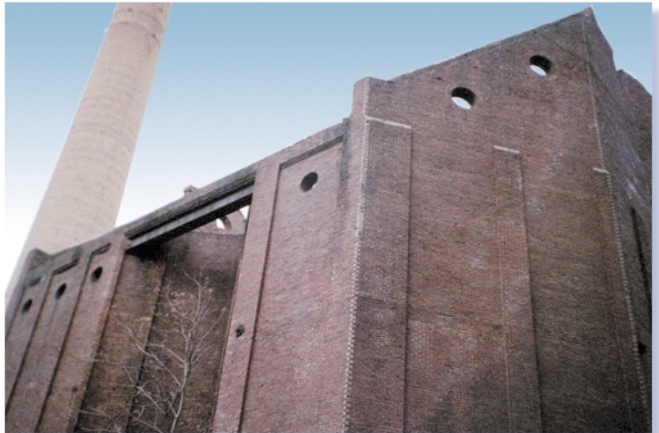
This coal house, built in 1899, is part of the Assets Site, an EPA brownfields site in Lowell, Massachusetts, where Volpe staff are performing an environmental site assessment. The EPA Brownfields Initiative helps revitalize urban areas by supporting the cleanup and sustainable redevelopment of contaminated industrial sites.
