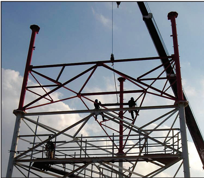
Iraqi tower construction. (Volpe Project File)
