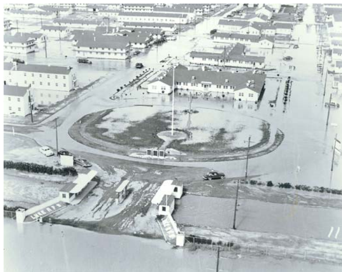
Flooded Front Gate
