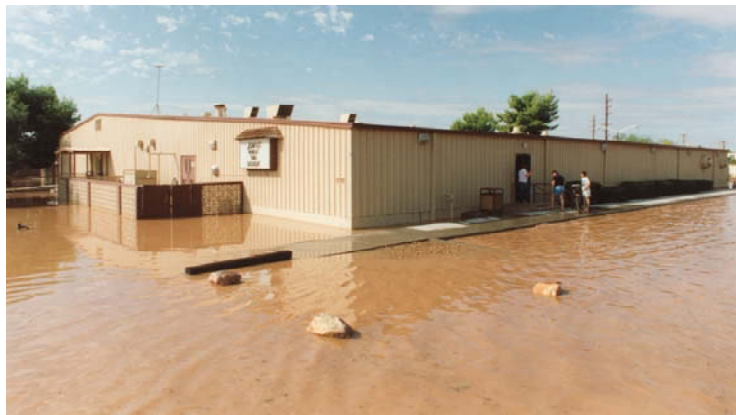
Flooded Base Bowling Alley, 20 October 1992
