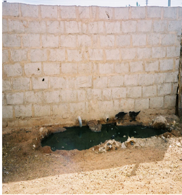
Photograph of poor drainage next to the side of a house, Marawa, Jigawa (December 2004)
