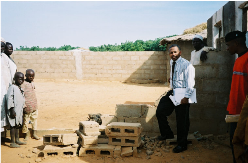
Photograph of a crumbling wall within the compound of houses, Marawa, Jigawa (December 2004)
