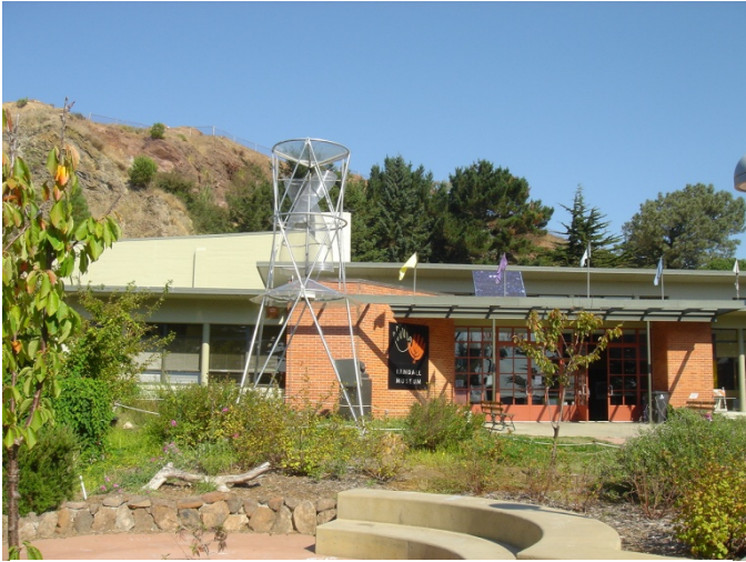
Figure 20. This Aeroturbine at the Randall Museum in San Francisco, California, is an example of a vertical-axis wind turbine in the built environment. Photo from Danielle Murray, Department of the Environment, San Francisco, NREL/PIX 18443
