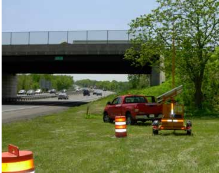
Figure 7. Wavetronix Trailer During Data Collection Setup
