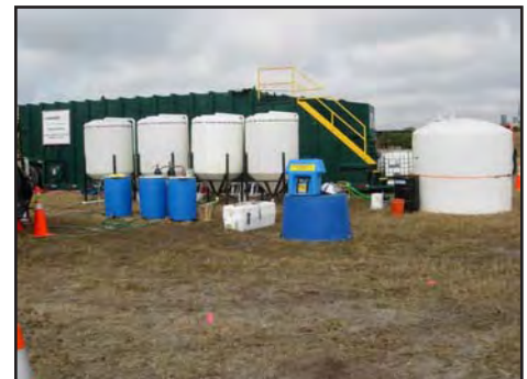
Figure 2. Photo of mixing and injection setup.
