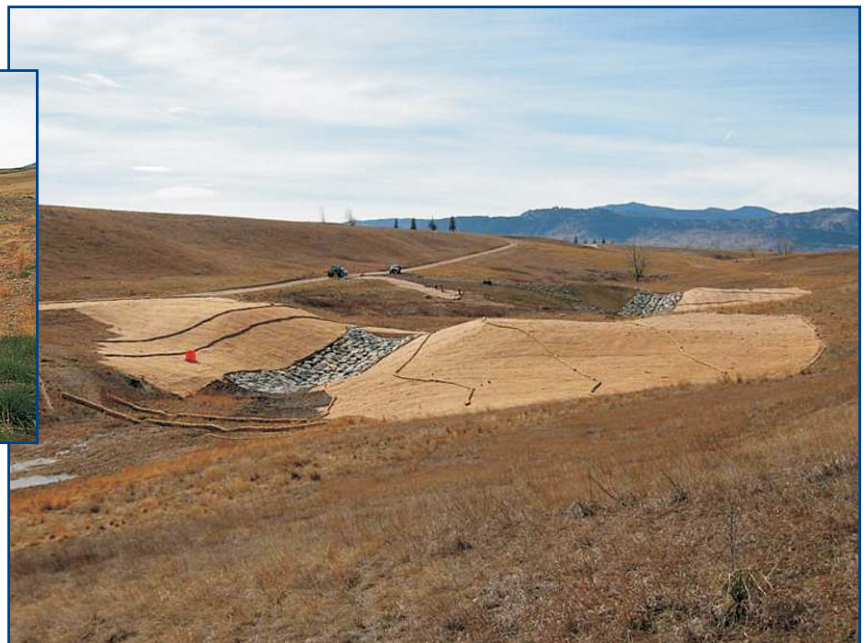
Rocky Flats dam B-2 following project completion.
