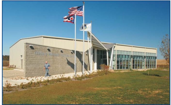
The high-efficiency windows in the Office of Legacy Management's Fernald Preserve Visitors Center provide natural light and passive solar heating. A green building also offers environmental, economic, health, and community benefits.
