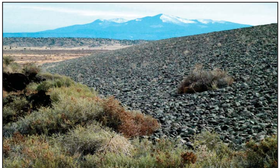
The Bluewater UMRCA Title II disposal site is in the Grants Mineral Belt of New Mexico. The main cell at Bluewater is the largest UMRCA cell managed by LM, covering over 400 acres (162 hectares). Mt. Taylor, a prominent peak in western New Mexico, is in the background.
