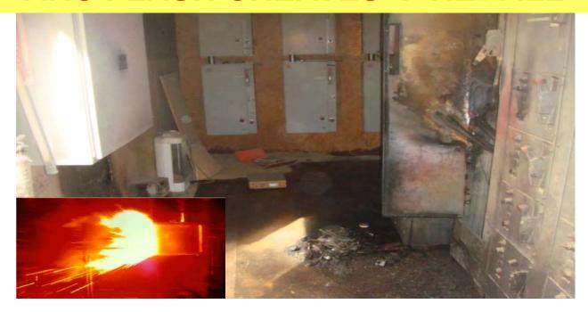
An electrical accident occurred on October 10, 2010, that caused the death of one contract electrician and seriously injured two coworkers. They were installing ground fault indicator lights in a circuit breaker enclosure when an arc flash occurred. They were not aware the circuit breaker enclosure contained a bottom feed circuit breaker and had locked out the wrong disconnect switch.
