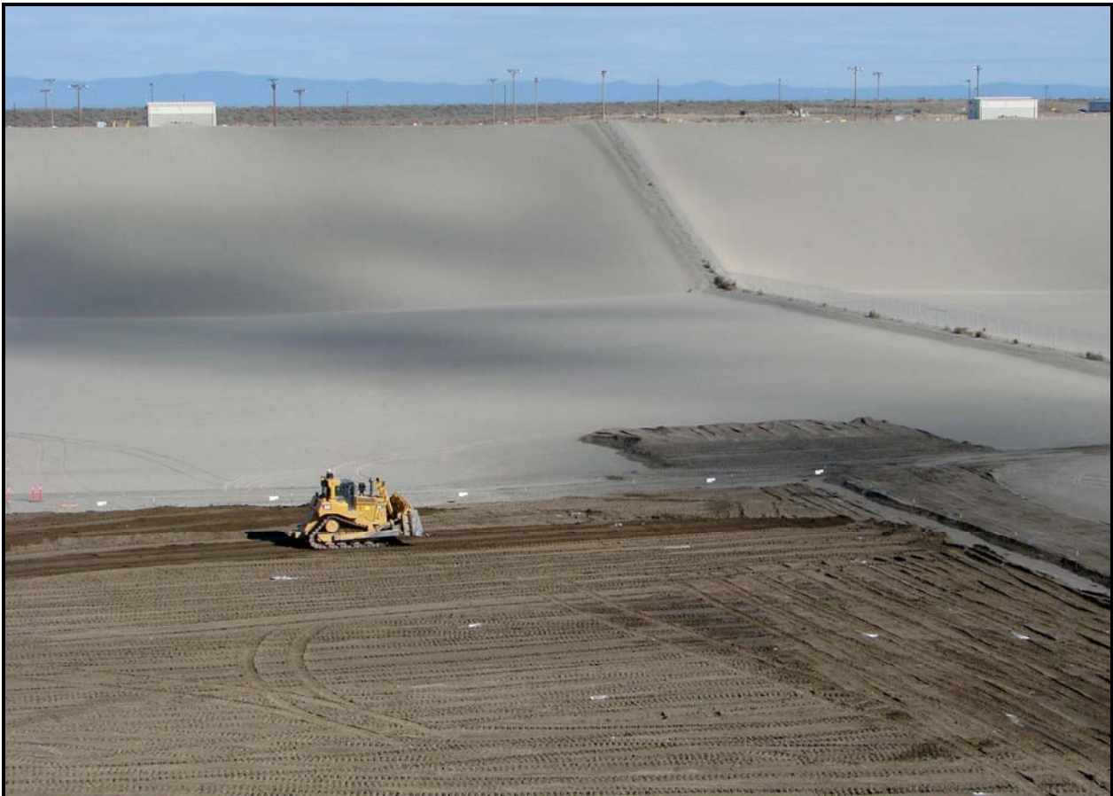
Waste is spread across super cell 9 at the Environmental Restoration Disposal Facility. The super cell was placed into service in mid-February. (Photo 1)
