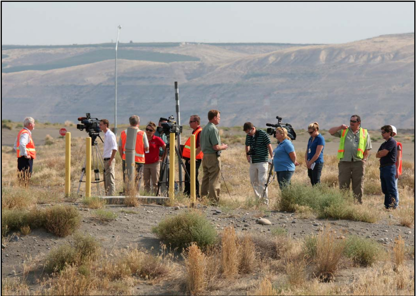
Representatives of the U.S. Department of Energy's Richland Operations Office and Washington Closure Hanford brief local reporters on intrusive characterization activities at the 618-10 Burial Ground.
