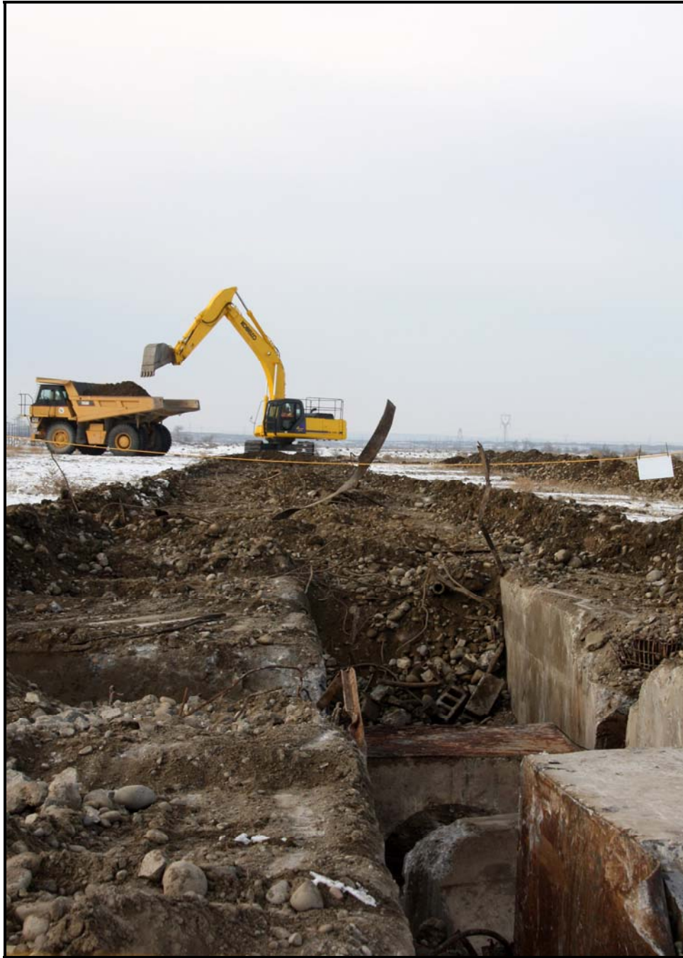
Washington Closure Hanford subcontractor Ojeda Business Ventures performs remediation activities at 100-F-57, the former site of a water treatment plant with buried pipeline and cradles. (Photo 8)
