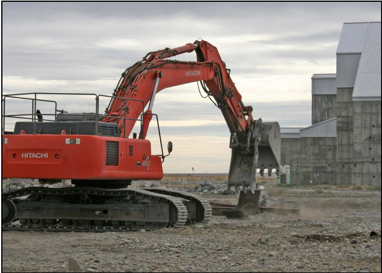
Ojeda removes debris from 100-F-57 during excavation. (Photo 5)
