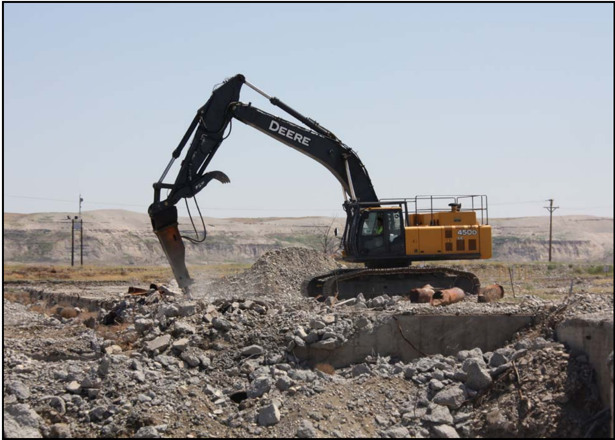
Ojeda Business Ventures continues to demolish concrete at site 100-F-57. (Photo 8)
