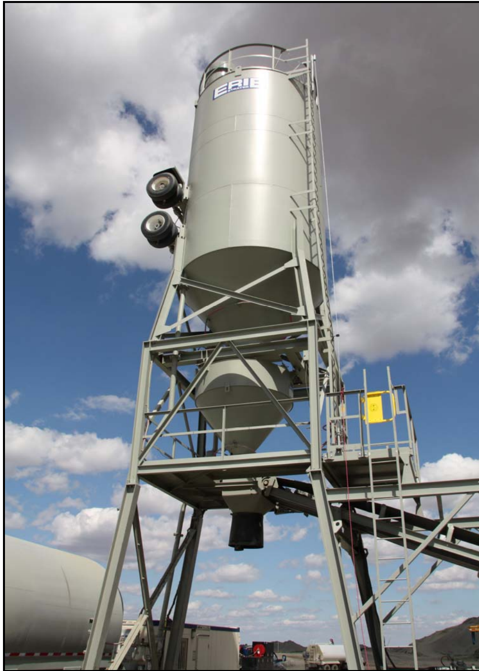
ERDF's new batch plant will manufacture concrete used to mix with debris, ensuring no void space during disposal operations. (Photo 4)
