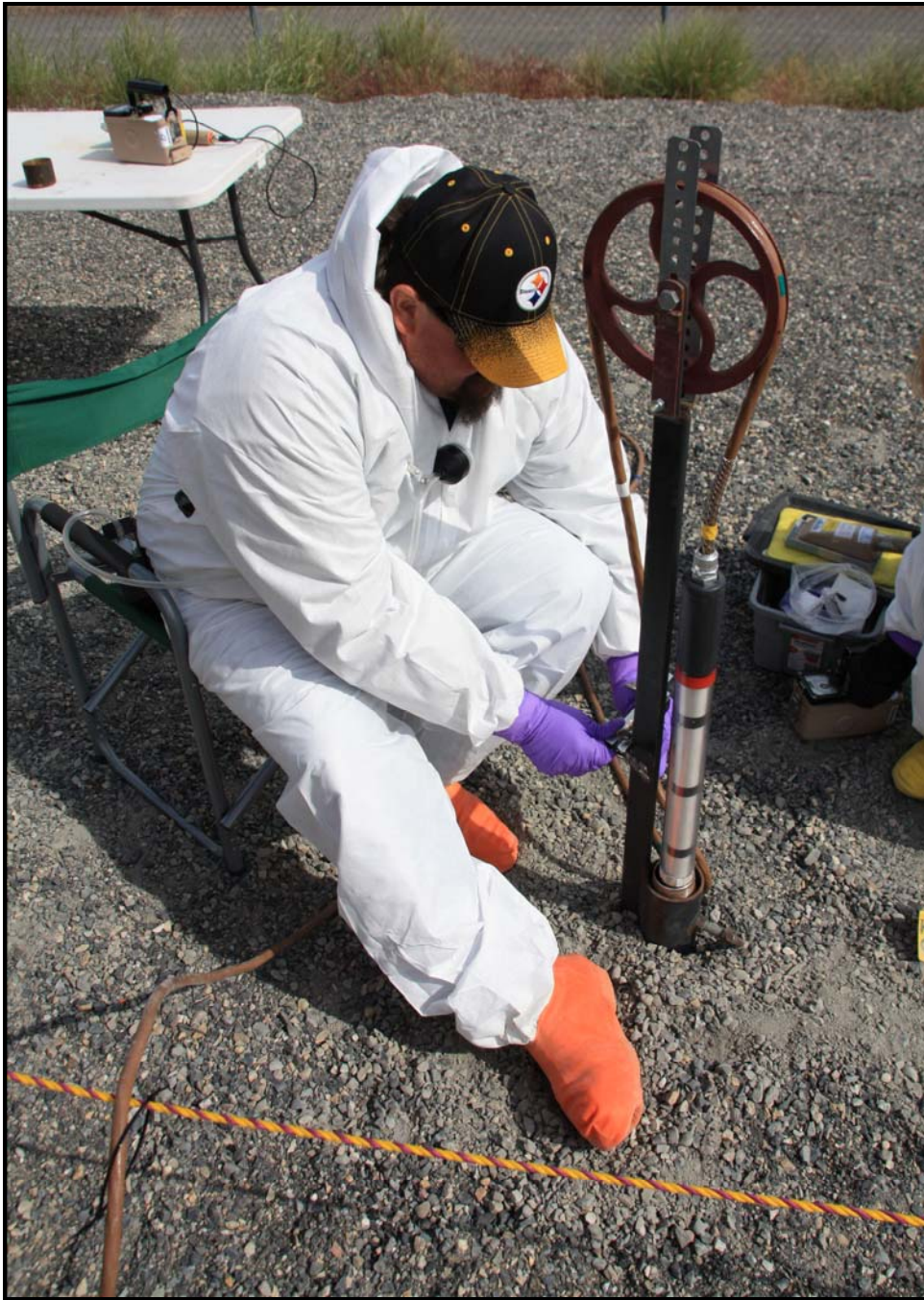
An employee with Washington Closure Hanford subcontractor North Wind lowers a multi-detector probe into a cone penetrometer at the 618-11 Burial Ground. (Photo 7)
