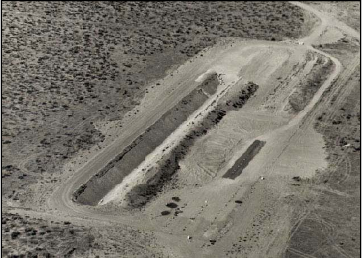
One of the three slope-sided trenches at the 618-11 Burial Ground. (Photo 7)
