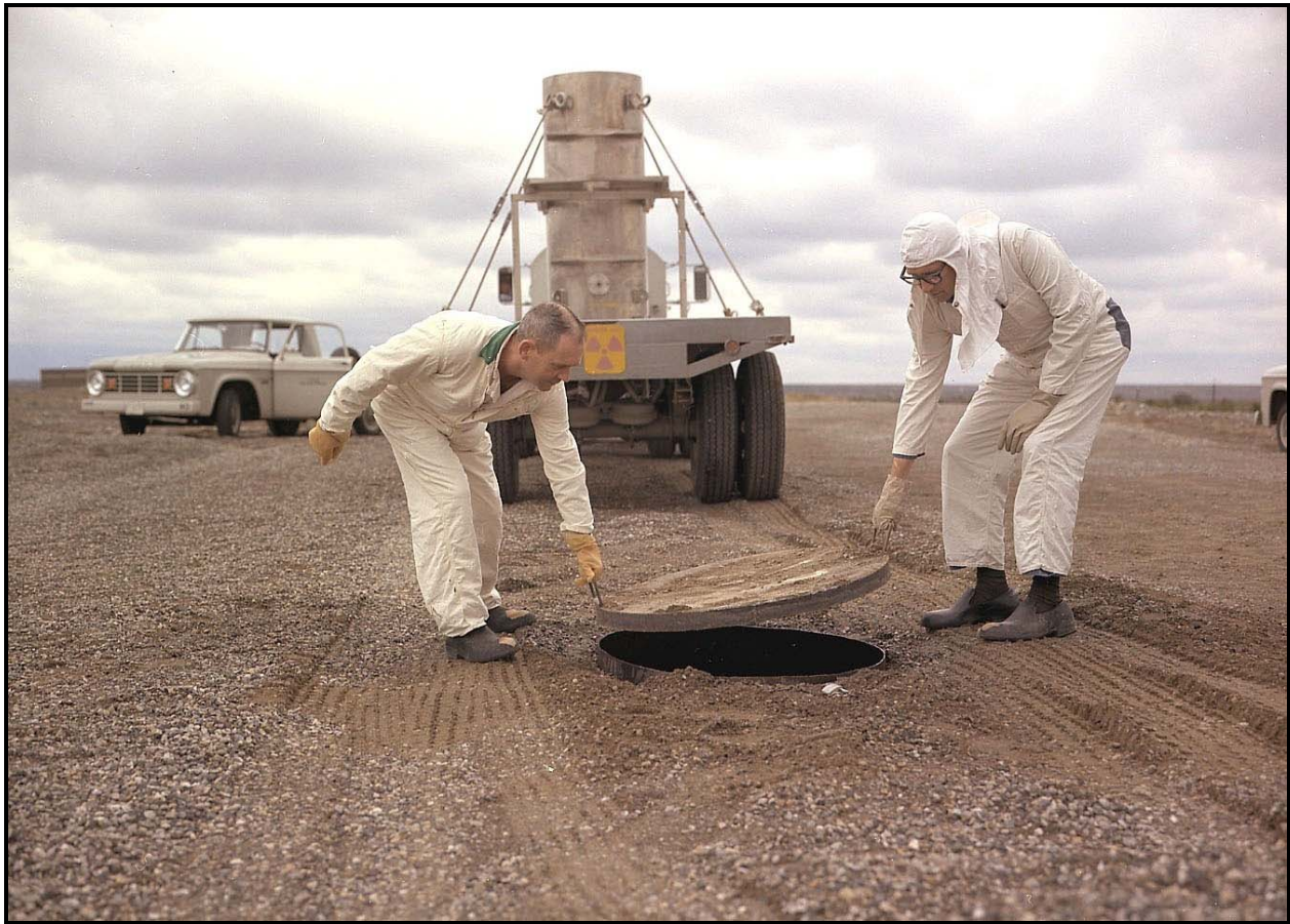
This April 1967 photo shows Workers placing the cover over a caisson at the 618-11 Burial Ground. (Photo 8)
