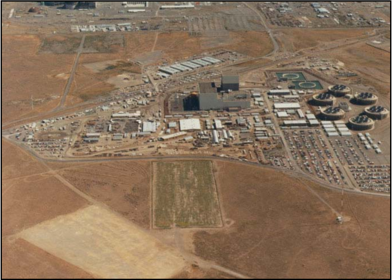
In this July 1998 photo, the green rectangle is the 618-11 Burial Ground. The site is adjacent to the Columbia Generating Station, a commercial nuclear plant. (Photo 7)
