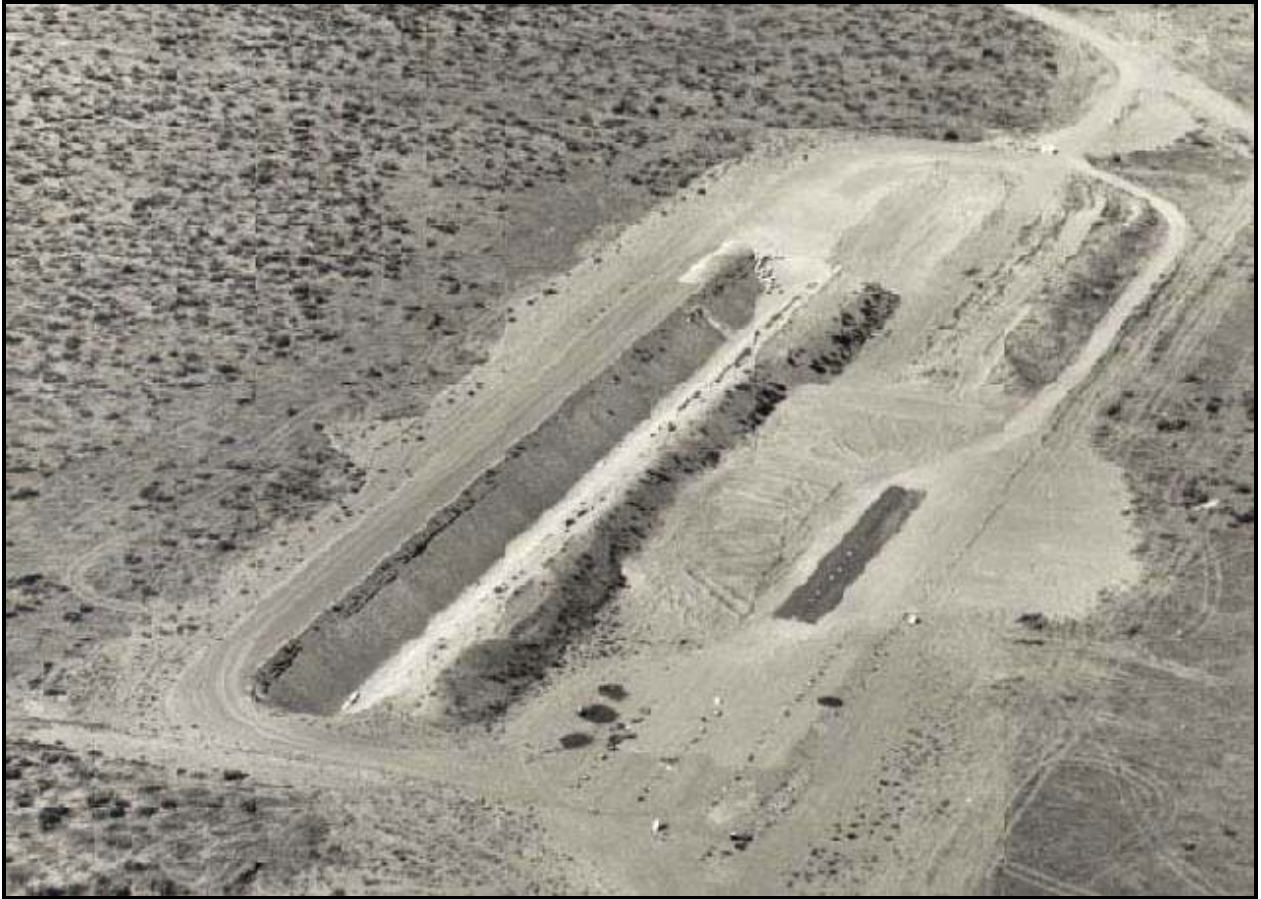
This August 1964 photo shows an open trench at the 618-11 Burial Ground. Caissons are visible in the lower right corner and right side of the photo. (Photo 8)
