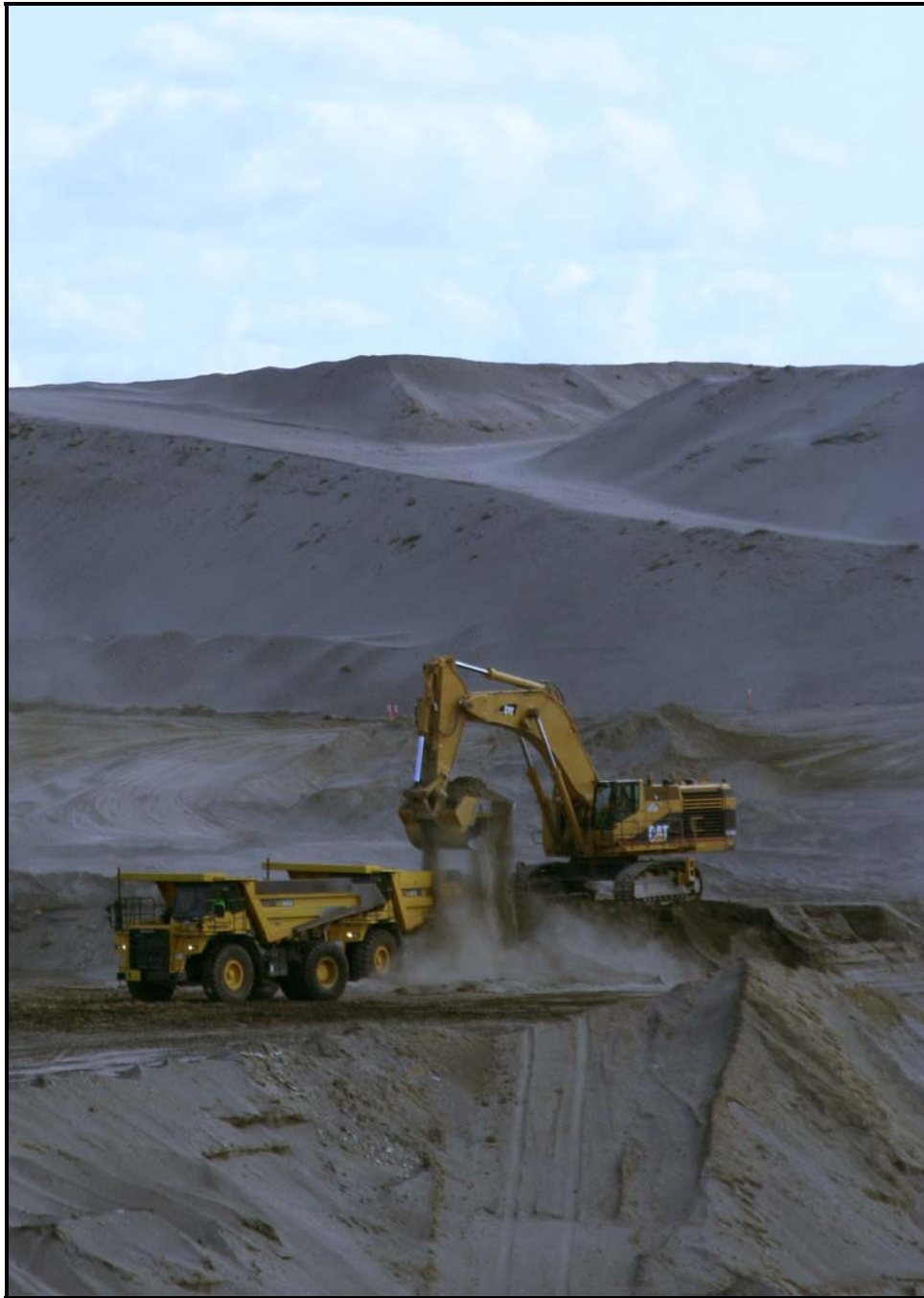
Work continues at super cell 10 at the Environmental Restoration Disposal Facility.
