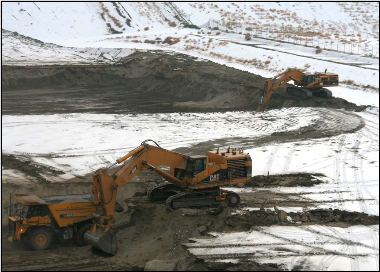
More than 80 percent of the dirt has been removed from super cell 9 at the Environmental Restoration Disposal Facility.
