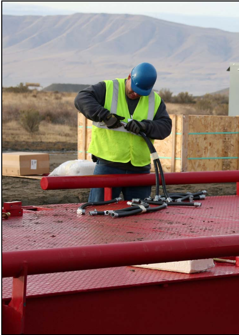
Installation of the new scale at ERDF nears completion.
