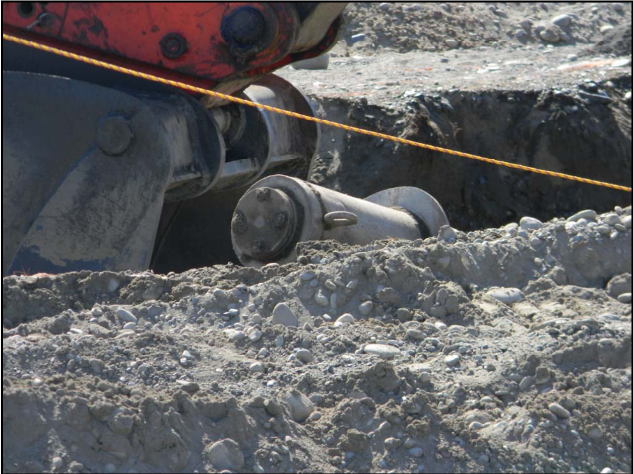
A shipping cask was discovered during cross-trenching of the 618-10-1 trench at the 618-10 Burial Ground.
