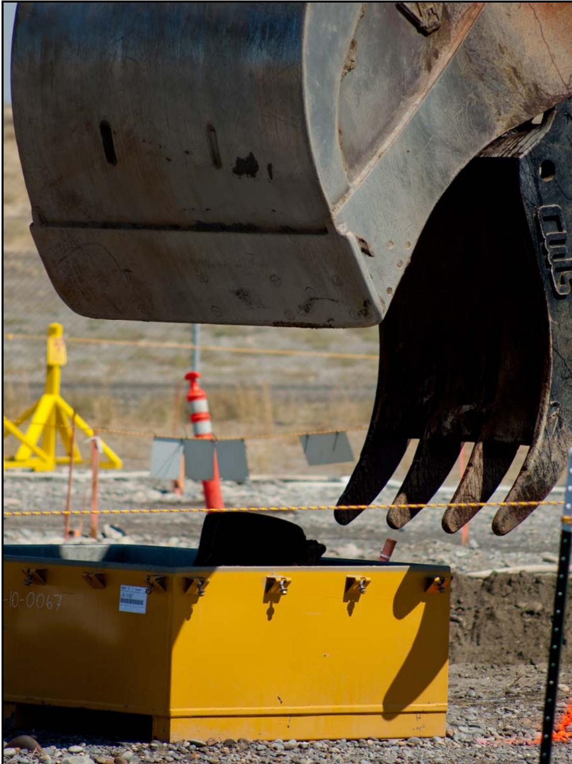
The unearthed drum discovered at the 618-10 Burial Ground was confirmed to contain depleted uranium chips in oil.
