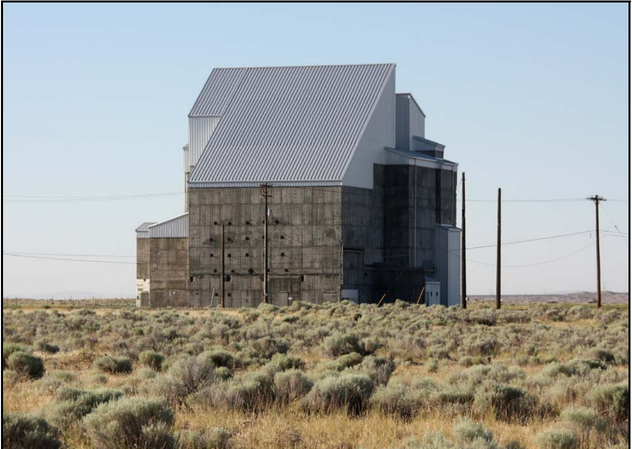
F Reactor was the third of Hanford's three original nuclear reactors. It was cocooned in 2003, making it the third Hanford reactor to have its core encased in a concrete shell.
