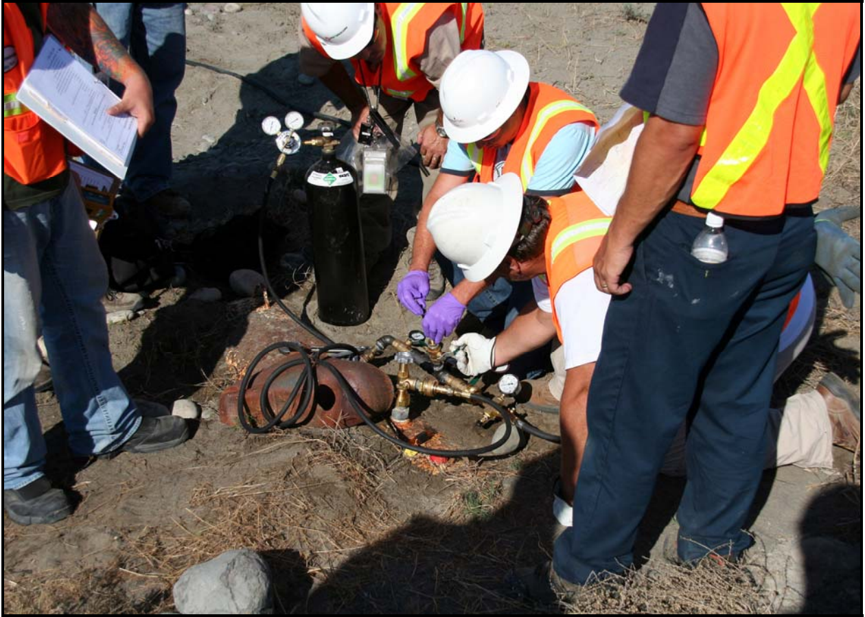
Washington Closure Hanford employees take a sample of the buried tank at the 618-10 Burial Ground. The tank was confirmed to have contained propane in the past.
