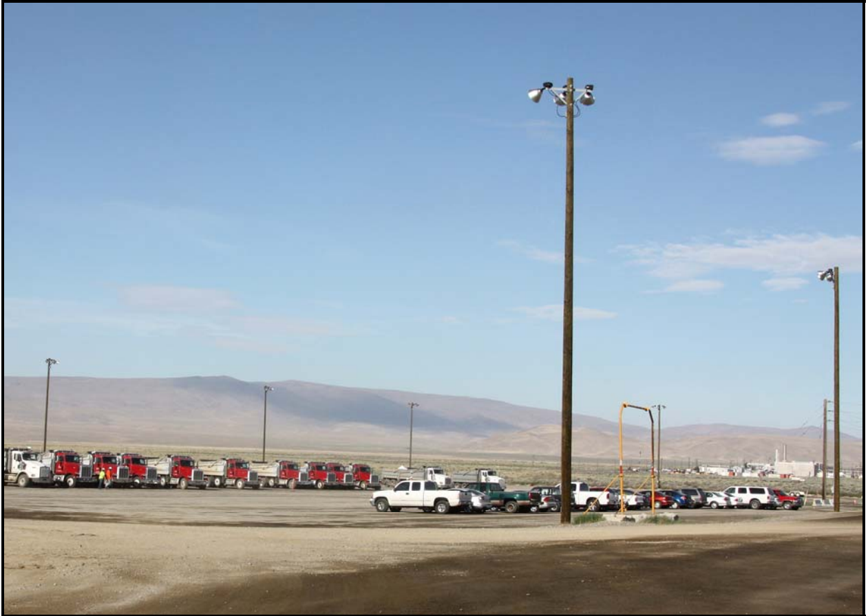
Washington Closure Hanford subcontractor George A. Grant has erected 15 light posts in the Environmental Restoration Disposal facility's transportation yard.
