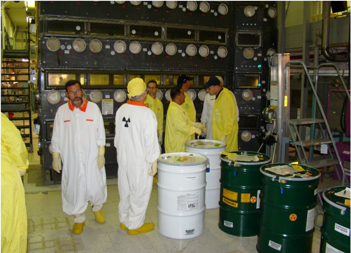
The fieldwork team performs a walk down as part of the job hazard analysis for cleanout of the HA-28 conveyor. The walk down supports the work control document for isolating the conveyor's utility systems and removing internal equipment in order to start chemical decontamination of the internal surfaces. The conveyor is connected to several glove boxes in Room 235B, including the four-level HA23S glove box shown in the background, which will also be removed with the support of Recovery Act funds.
