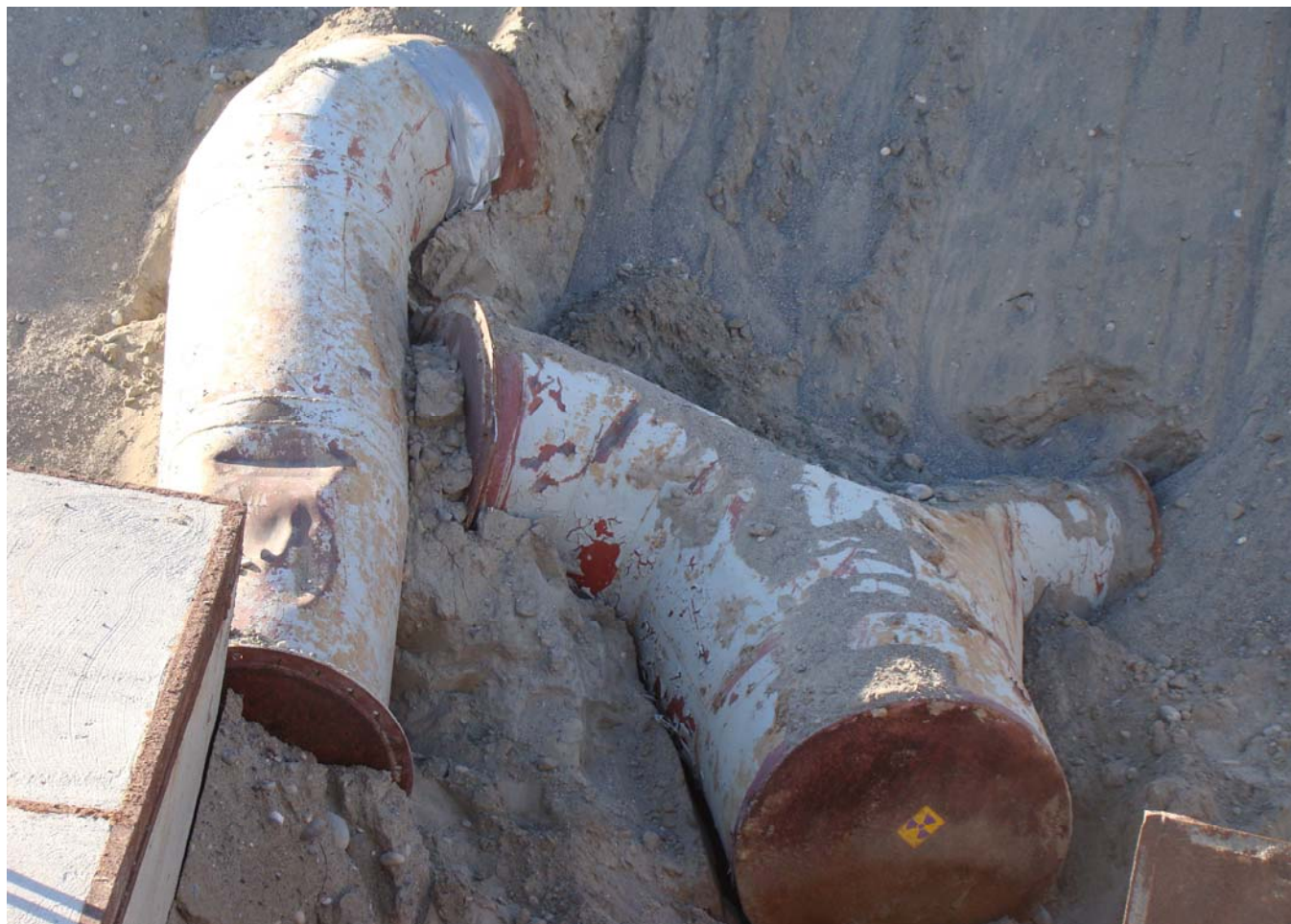
Two-foot diameter duct sections that have yet to be removed from 218-W - 4B Trench 11. These containers must undergo the same evaluation process as other standard waste containers but may require different overpacks to accommodate their abnormal shape.
