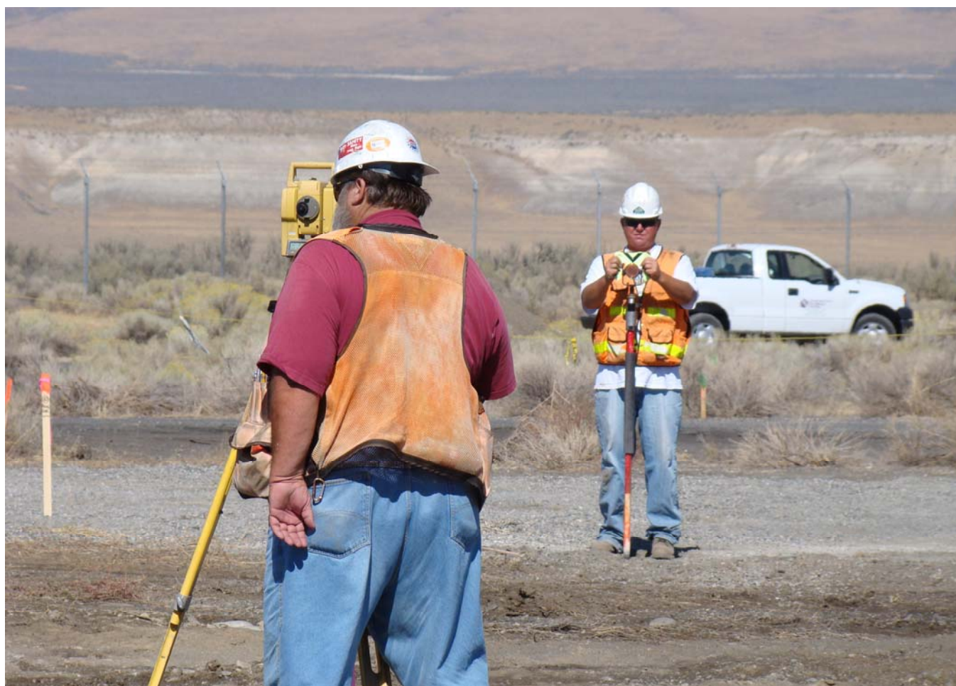
Workers stake the boundary for the DX groundwater treatment facility, which is one of two pump-and-treat systems that will be constructed with funds from the Recovery Act.
