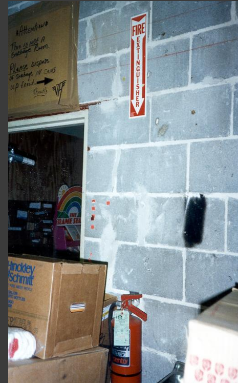
Blocked extinguisher
