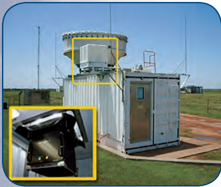
The WACR provides improved sensitivity for detecting tiny objects in the atmosphere to an altitude of 5 km. The instrument's antenna is located adjacent to the MMCR antenna on top of the MMCR shelter; the rest of the unit is located inside (inset).
