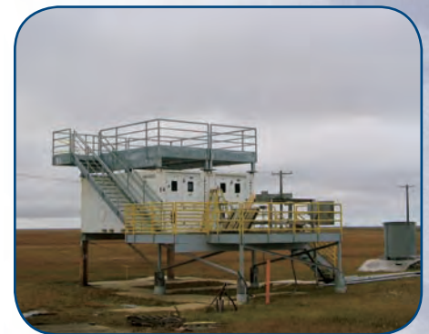
In September, installation was completed on the new Guest Instrument Facility in Barrow to provide additional instrument space and ease crowded working conditions.
