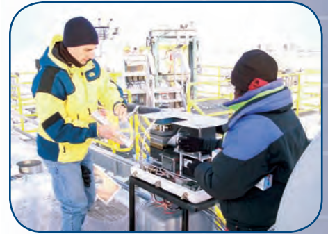
The 183 GHz radiometer, protected inside an insulated enclosure (inset), is installed on the roof of the primary instrument shelter at Barrow. To prevent snow from accumulating on the mylar window, a blower mounted beneath the radiometer directs air through a duct to a standard Y-shaped fitting mounted on top of the radiometer.
