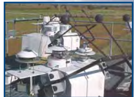
Pyranometers mounted on an automatic solar tracker, equipped with a shade mechanism to block the direct solar rays, provide measurements of diffuse irradiance.
