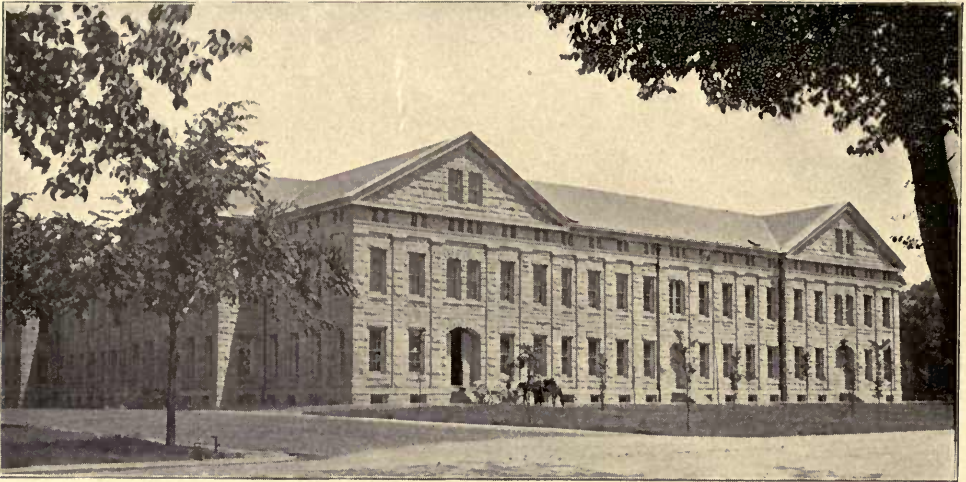
SHOP K. TYPICAL OF THE EIGHT REGULAR SHOPS.
