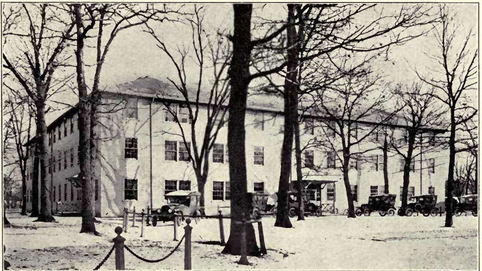
Temporary Office Building No. 2. It was necessary to provide quarters for hundreds of extra office workers during the war. This is one of the buildings erected for that purpose.
