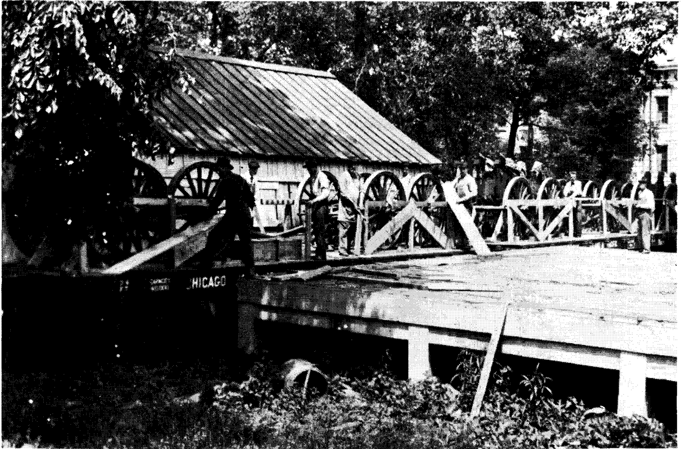
Below: RIA employees loading artillery carriages, 1898, shop A, (building 102) in background, looking northeast. The carriages final destination was Cuba to be used in support of U.S. troops engaged in the Spanish-American War.
