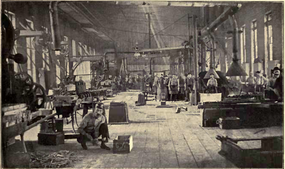
THE MAIN BLACKSMITH SHOP—INTERIOR.
