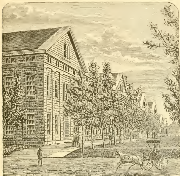
PARTIAL VIEW OF ARMORY SHOPS.
