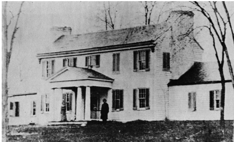
Davenport House built in 1833. (Picture taken from Reference 13 – page 46)
