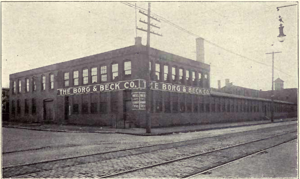
The Moline Plant
