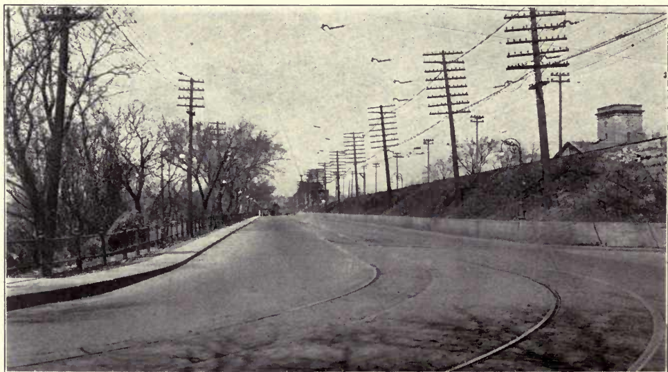
Fort Armstrong avenue. Public highway between bridges at west end of Island and sole traffic artery between Illinois and Iowa shores at this point.
