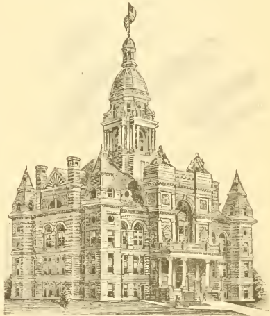
SCOTT COUNTY COURT HOUSE.
