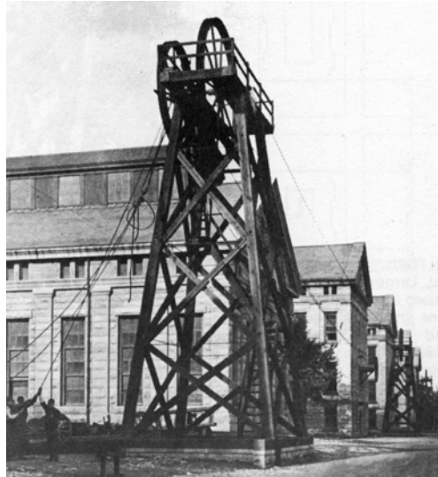
This is one of the towers holding pulleys that delivered the mechanical power from the hydropower dam to the Rock Island Arsenal shops shown in the background. (Picture taken from page 76 of reference 13)
