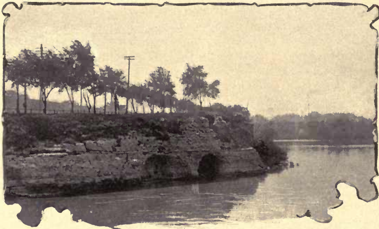
THE LOWER END OF ROCK ISLAND.
