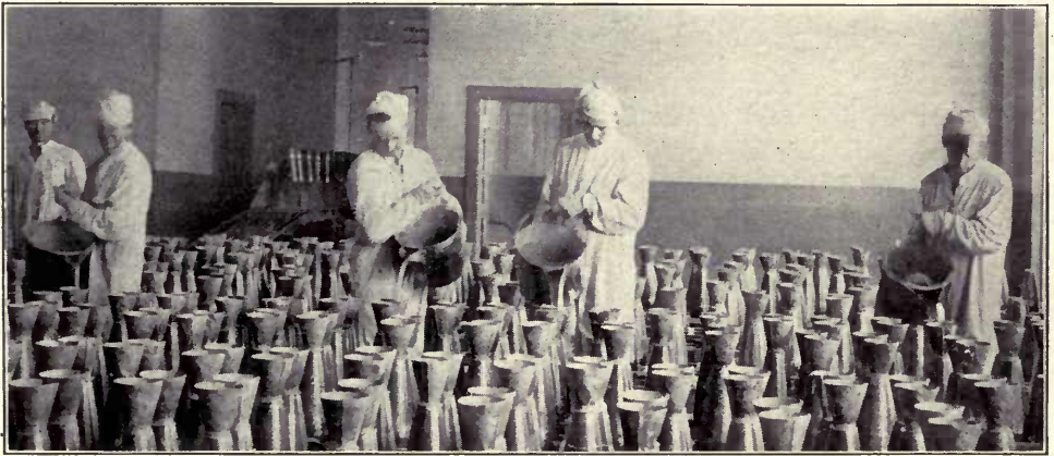
Bottling destruction in the form of molten trinitrotoluol, which is being poured into howitzer shells.
