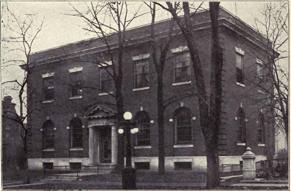
Rock Island Telephone Exchange.
