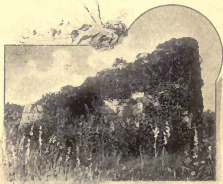
PIER OF THE FIRST BRIDGE.
