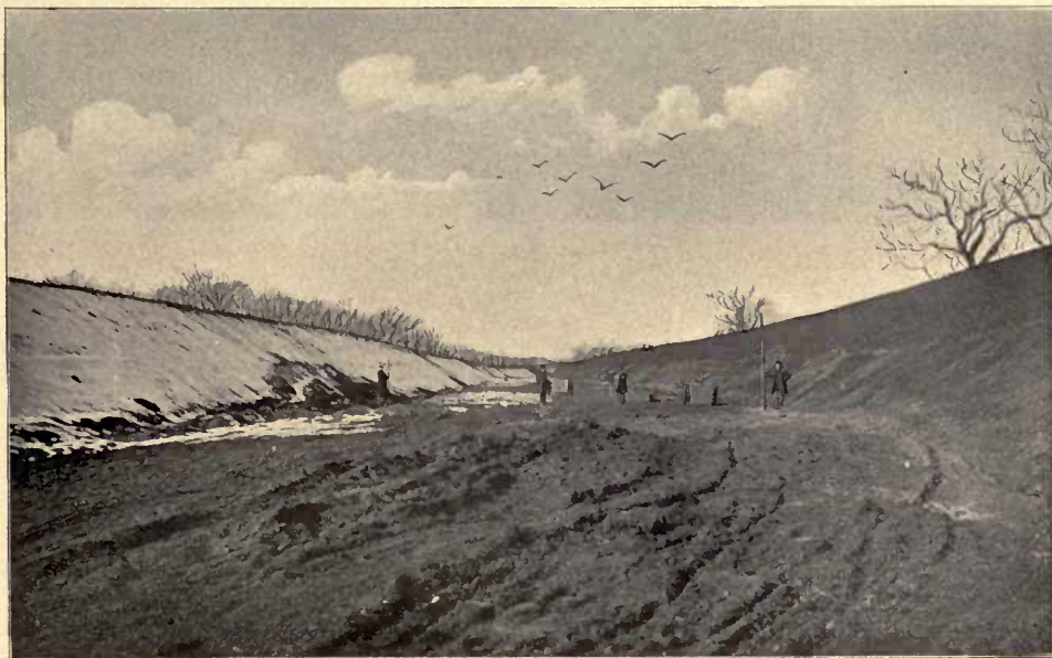
A SECTION OF THE CANAL READY FOR WATER.
