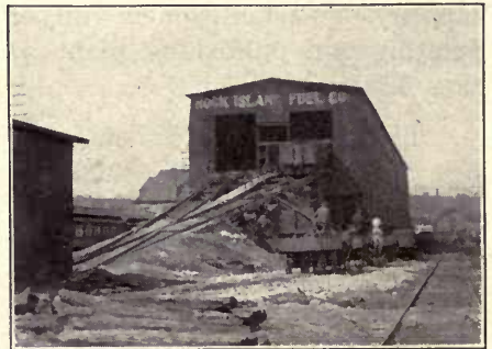
View of Gravity Bins
