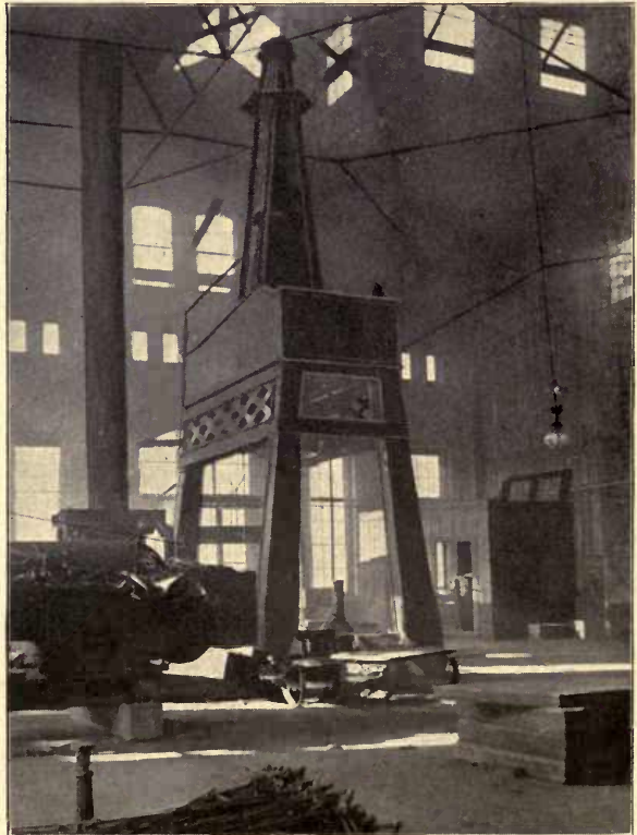
THE STEAM HAMMER.
