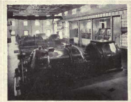
View of Power House Interior Showing Large Turbo-Generator Moline Ill.
