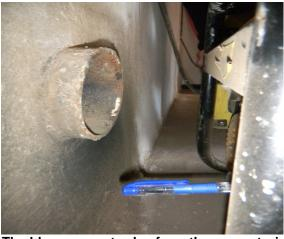
The blue pen protrudes from the generator's exhaust pipe to illustrate that the pipe does not align with the wall penetration on the left. (OIG photograph, September 9, 2011)
