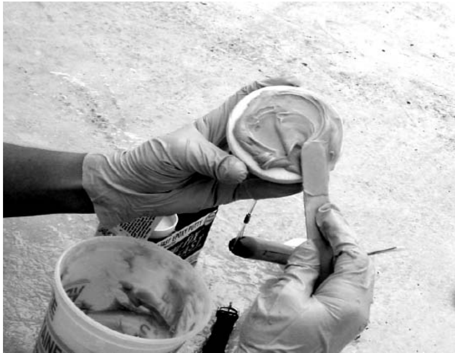
Figure 3: Applying the epoxy compound to PSAT baseplate.
